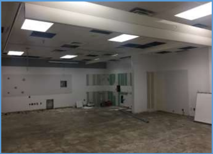
Wilson Middle School, Interior Demo, June 2018
