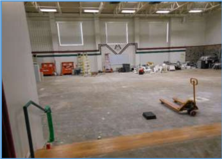
Miller Elementary School, Gym Demo, June, 2018
