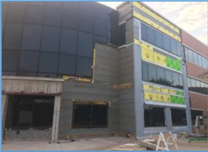
Academy High School Re-Brick, Mock-Up Wall, June 2017
