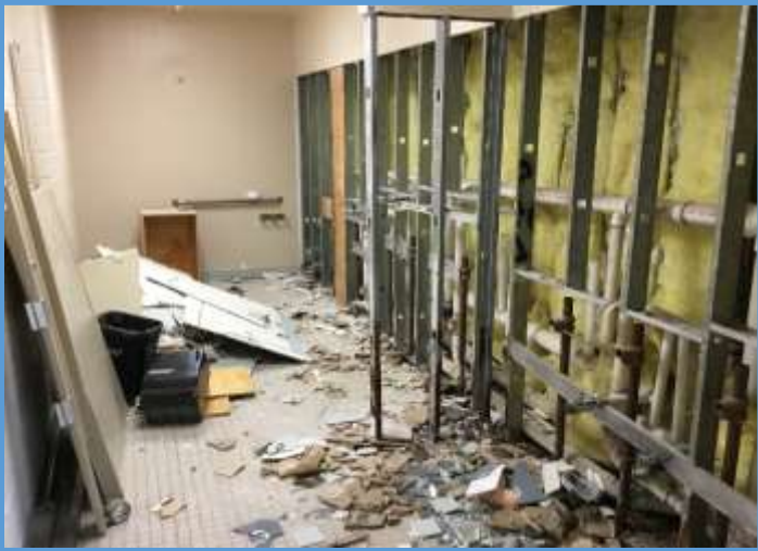
Jasper High School, Restroom Demo, June 2018
