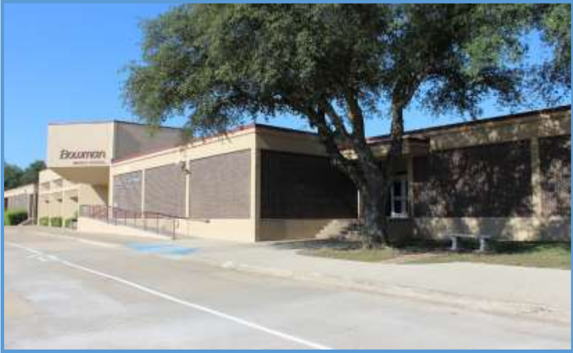
Bowman Middle School, Main Entry, June 2018
