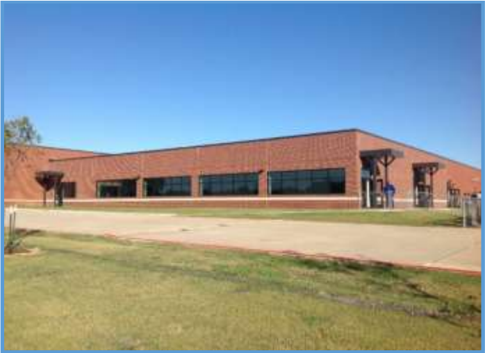
Guinn Special Programs Center, Classroom Addition, August 2017
