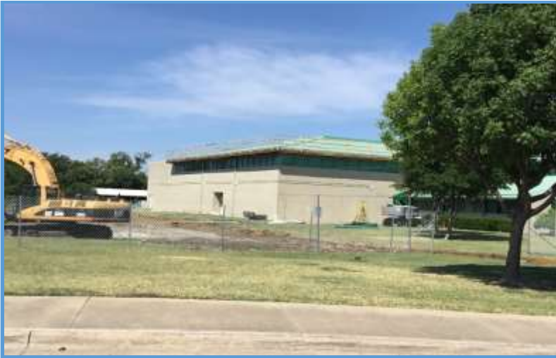
Robinson Middle School, Paving Removal, June 2018
