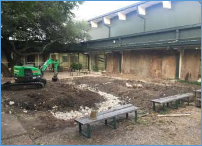
Wilson Middle School, Interior Courtyard Demo, June 2018
